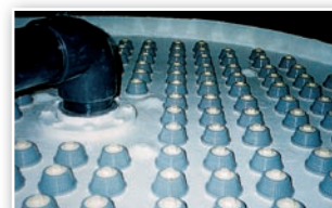
Fixed nozzle system
